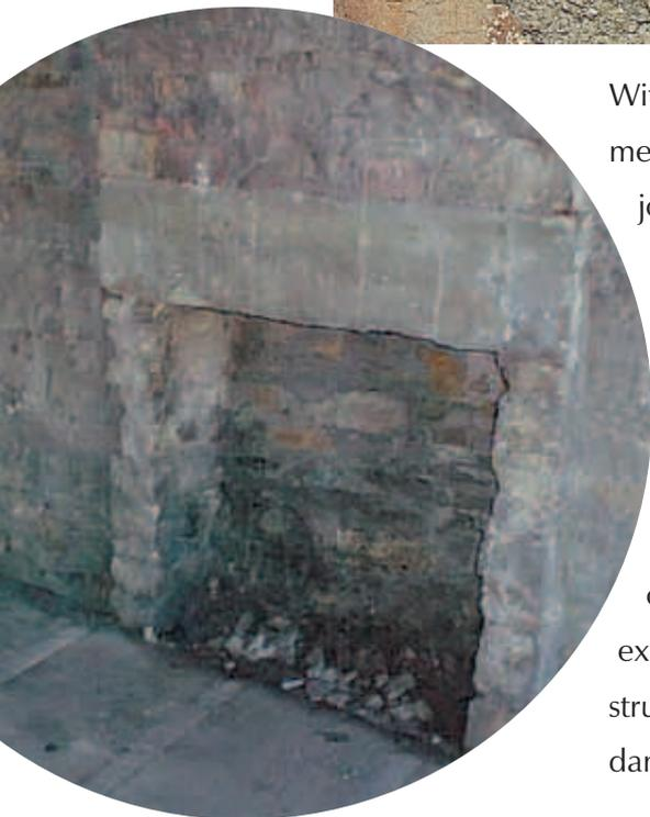
With the wall-cutting method the masonry is cut through mechanically and horizontal isolating material inserted into the joints. Injection methods require innumerable little drilled holes in order to chemically bring about an injection of the walling.
